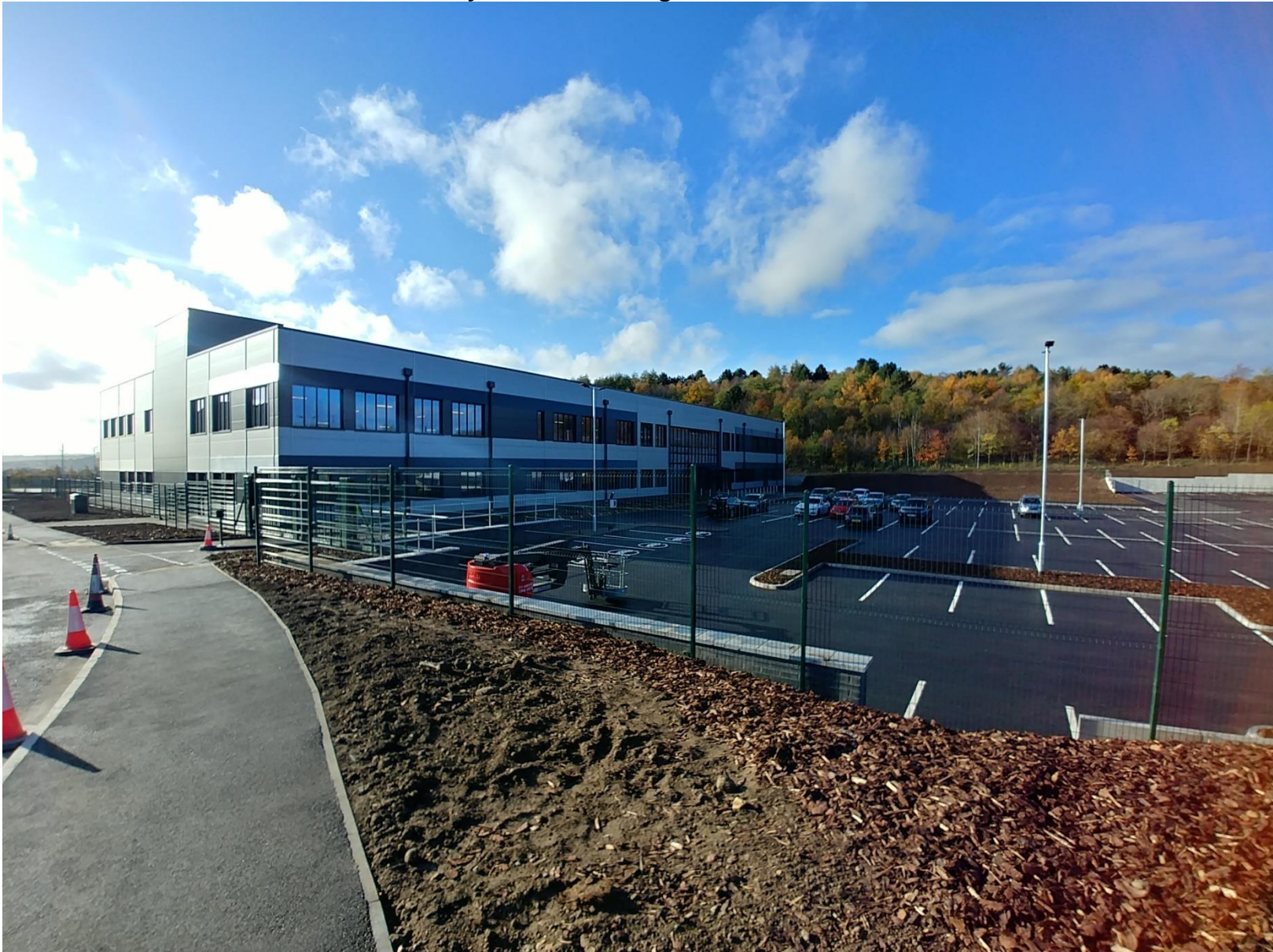
The new Barnsley Centre building – as handed over to NSHBT
